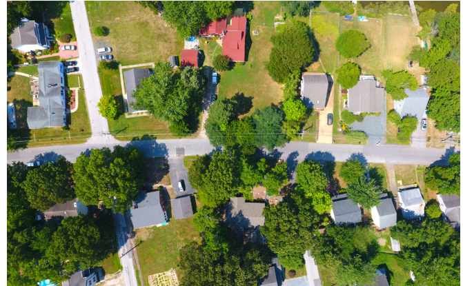
Anne Arundel County, Sewage Pump Station Force Main
